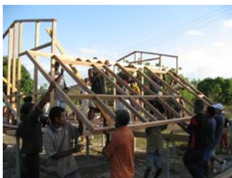
Building a GK house in Gerehu Stage 6
